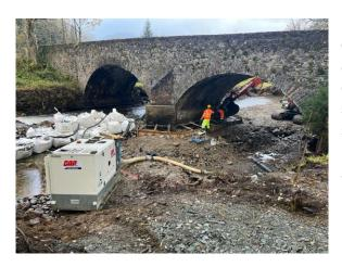
Emergency bridge works to deal with scour (water eroding damage the bridge abutment/foundation) been have completed and work is currently underway which stabilising the embankment, supports the road. There are a number of locations along the B828 where rock nailing and support beams are being installed.
