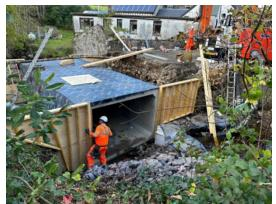
With the bridge and road now open to all traffic we have commenced work to carry out a hydrology study. This is a complex and technical piece of works which is required to design the training walls (the walls which direct the water flow into and out of the bridge structure), to satisfy SEPA in terms of retrospective consents and to ensure that the bridge will not have any adverse effect on the river. There is additional design work to carry
